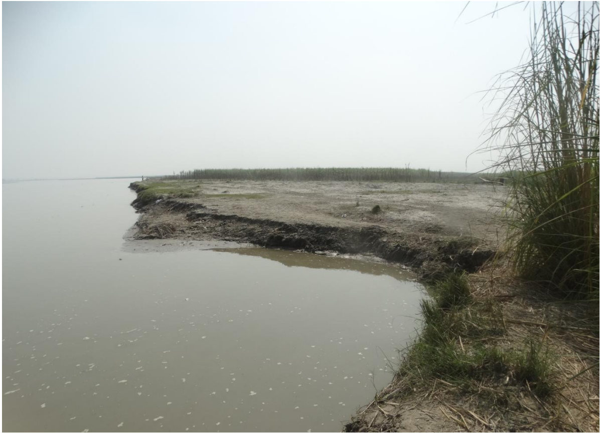
Image 25 : River Bank Erosion At Makhdumpur, Distt. Meerut
